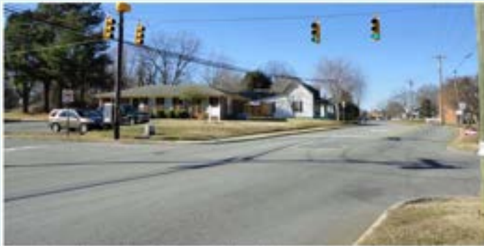
The majority of intersections in Gibsonville lack pedestrian crossing treatments, such as the intersection of Burlington Avenue and Apple Street shown above.
